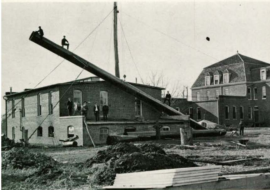
Preparations in 1910 for opening the school included the building of a furnace house and new boiler.
