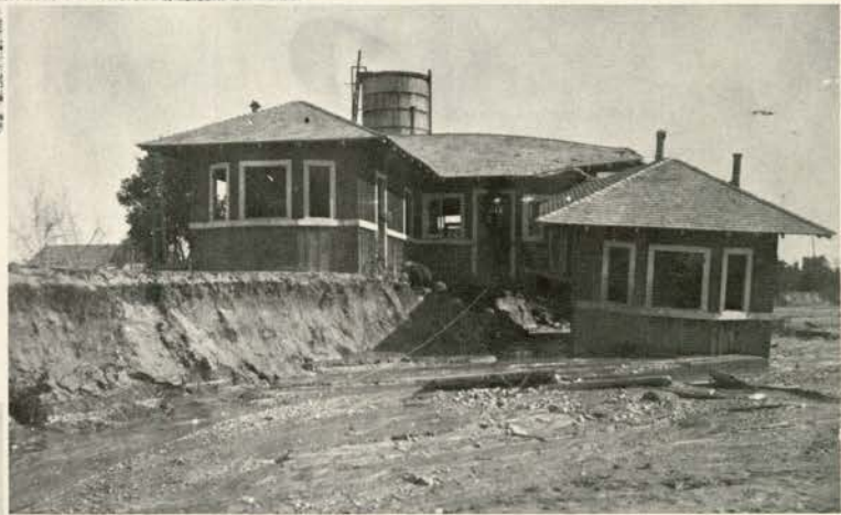
Below With the name of the house still fastened above the front door, the "Dew Drop Inn" became a favorite spectacle for people who came to view the devastation caused by the flood.
