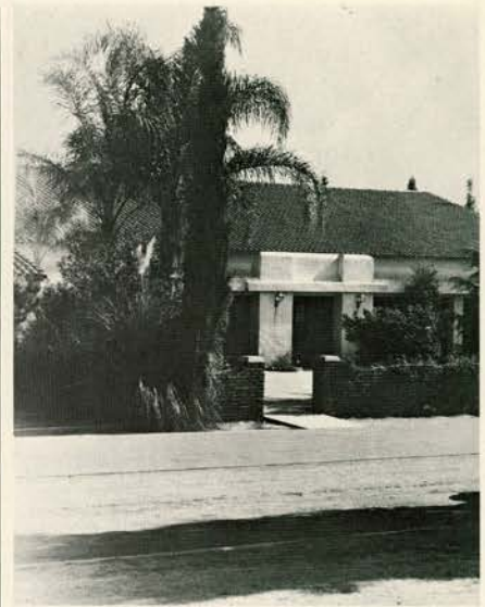
In 1941 the pride of both students and faculty was the addition of a food services building.
