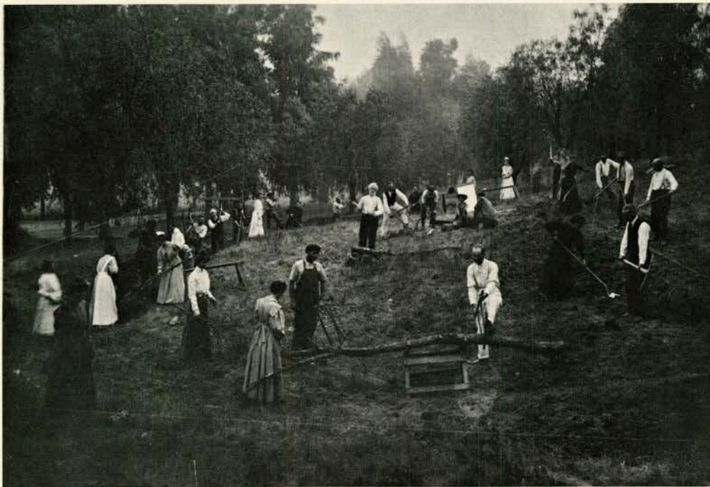
Left Ground breaking for the original Kate Lindsay Hall found both men and women out wielding picks and shovels to help get the project started.
