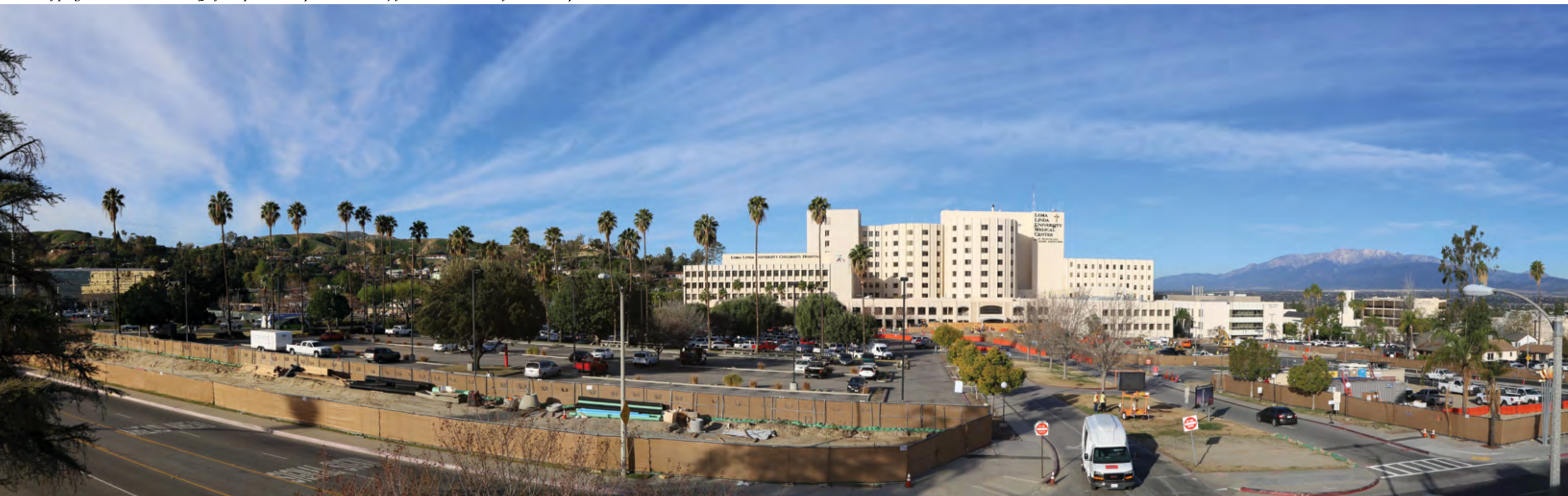
Below: With this excellent vantage point of the site for the new hospital towers from the Carroll S. Small Alumni Center, Alumni Association staff and visitors have already witnessed changes in the landscape over recent months and will continue to witness significant change over the next five years. The current entrance to the Medical Center, seen at bottom right, will soon give way to the hammer blows of progress as a new entrance off of Prospect Street opens to make way for the construction of the new hospitals.
