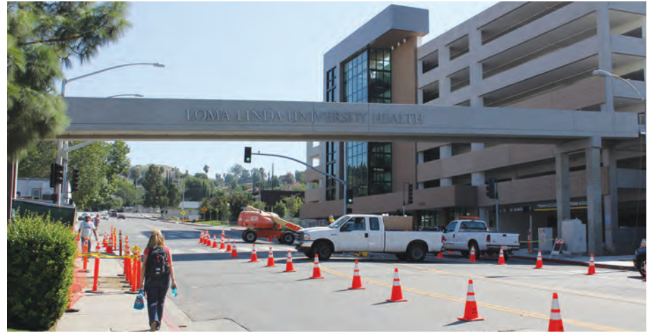
The Campus Street pedestrian bridge nears completion.
