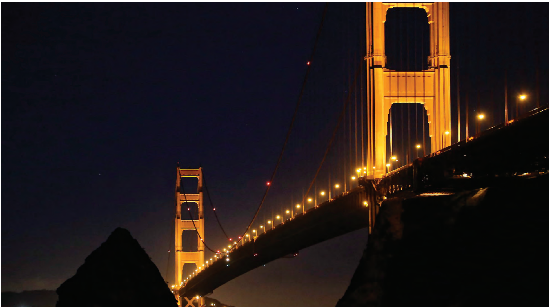
A view from below, Golden Gate Bridge
