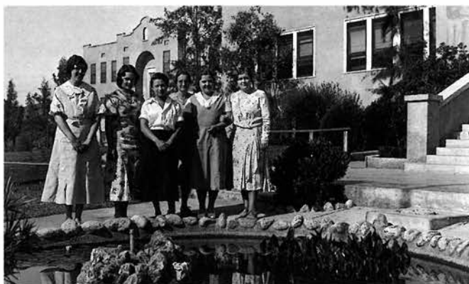
A pond once existed in front of La Sierra Hall
