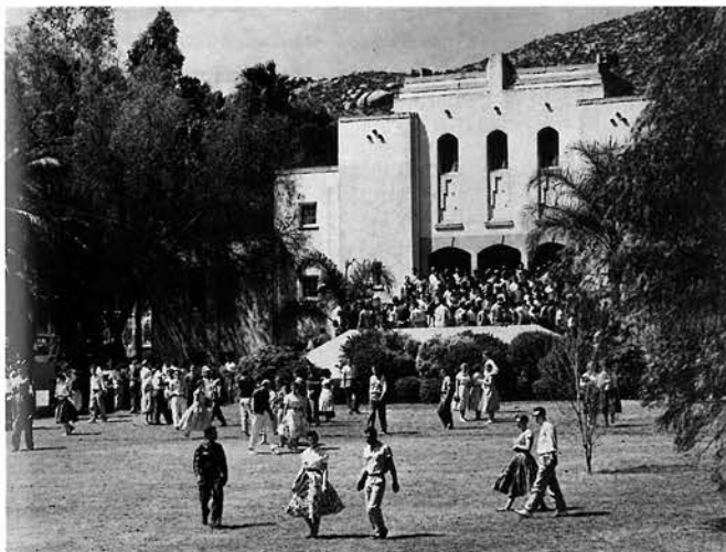
Hole Memorial Auditorium served as the location for chapel for many years as well as the location for the La Sierra Church for several years.
