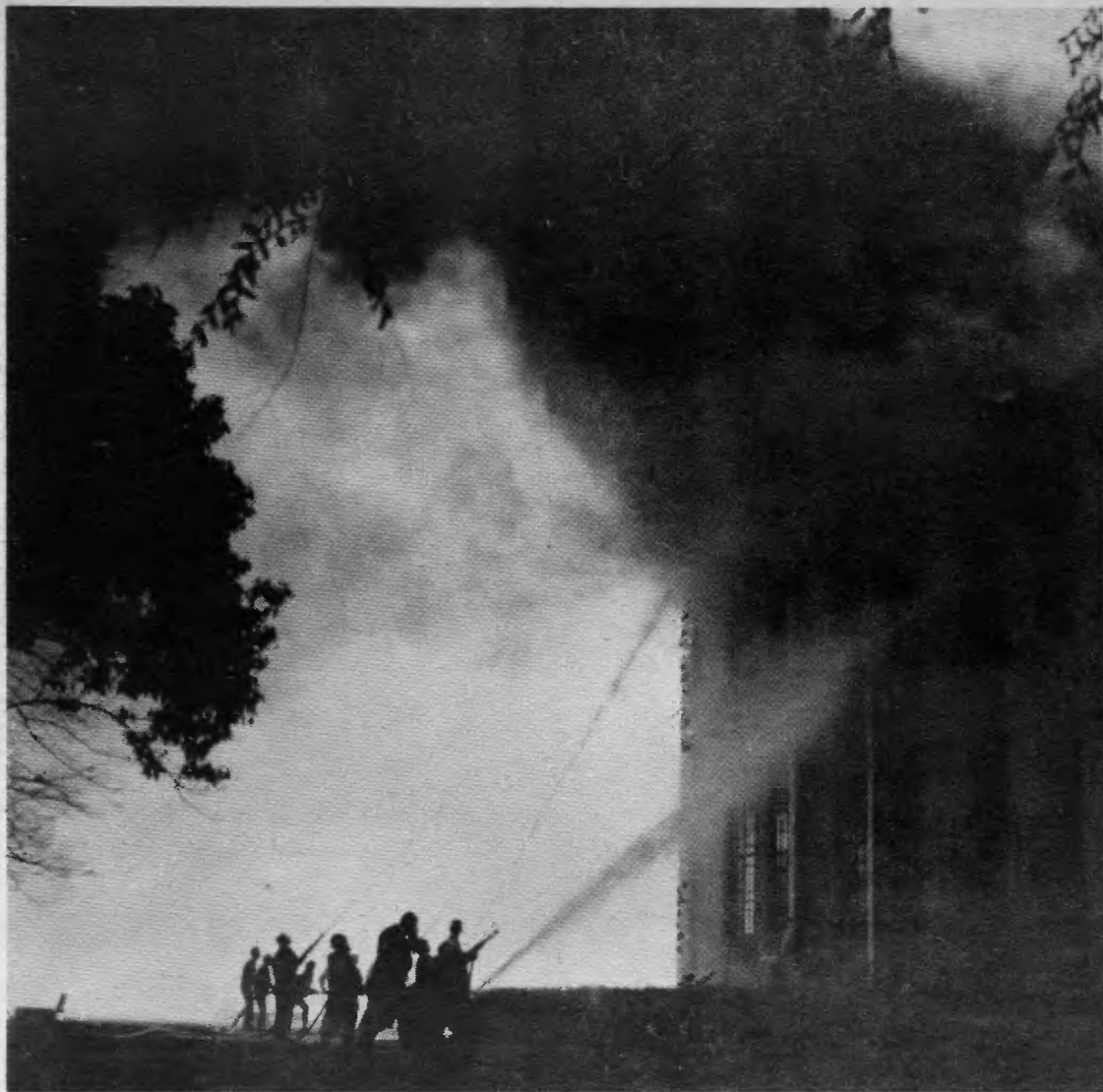
Firemen fight flames at east end of building.
