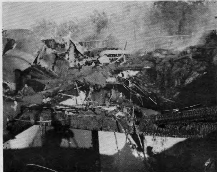
Entire third floor is reduced to charred rubble heap.
