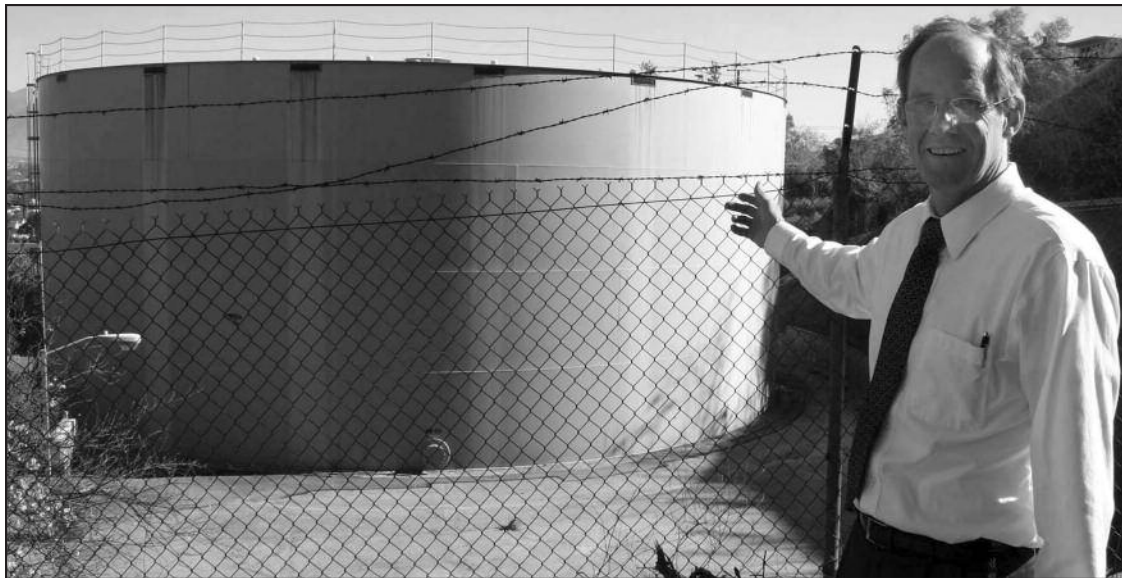
Ken Breyer, MA, assistant vice president for construction at LLUAHSC, points to one of two 1.4 million-gallon water towers on a hillside above Loma Linda. Despite the fact that Mr. Breyer is standing on a hillside at a location approximately three stories above ground level for the giant structure, its large dimension can be clearly seen. Even so, the new chilled water tower under construction on campus will be more than four times larger.
