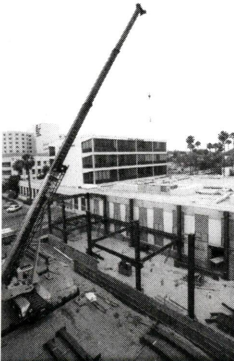
Prince Hall east addition's construction update: the steel girders forming the supports for walls and floors were installed starting May 19.
