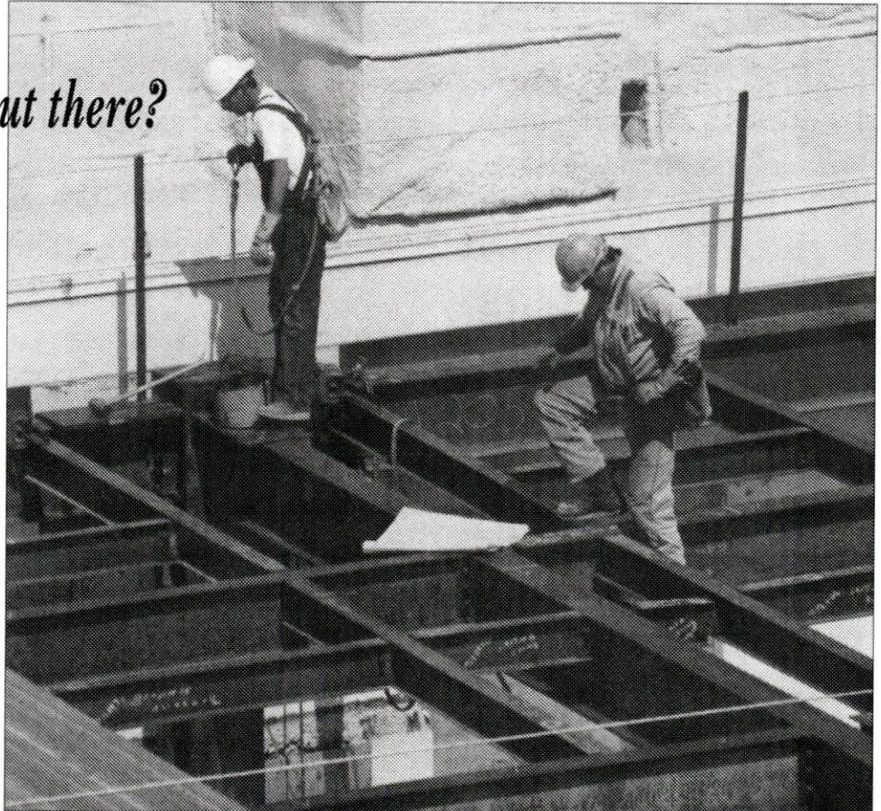
Prince Hall east addition's construction update: the steel girders forming the supports for walls and floors were installed starting May 19.
